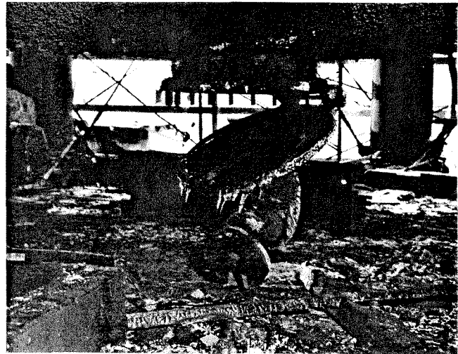
Figure 4. The fire started here underneath the sphere where a workman attempted to thaw out a frozen nozzle with a propane torch.
